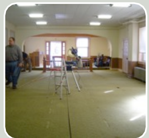
The Old Sanctuary at the beginning of the remodeling stage
